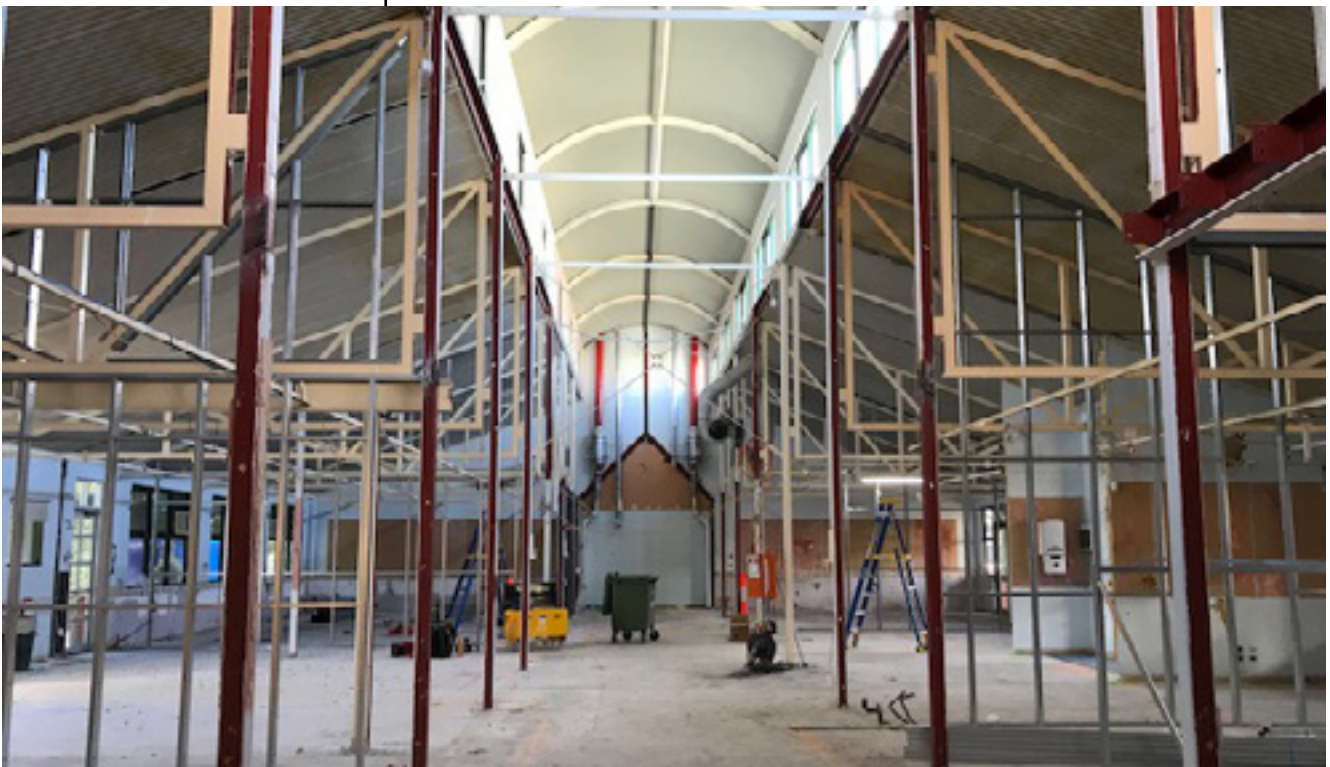
The new STEM area under construction
